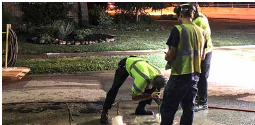
Pictured above is Lakewood Service Crew’s infamous Water Whisperer, who can find leaks just listening to the flow of water at the end of a long steel rod. Another great thing in Lakewood, our Service Crews! Fixed in hours, not days! Thank you!
