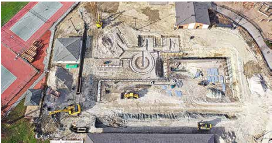
The Foster Pool Improvements project is well underway. The demolition is complete and underground utilities are currently being installed. The new pool layout is starting to take shape with the foundations, buttresses, and the pool walls being constructed under ideal weather conditions.
