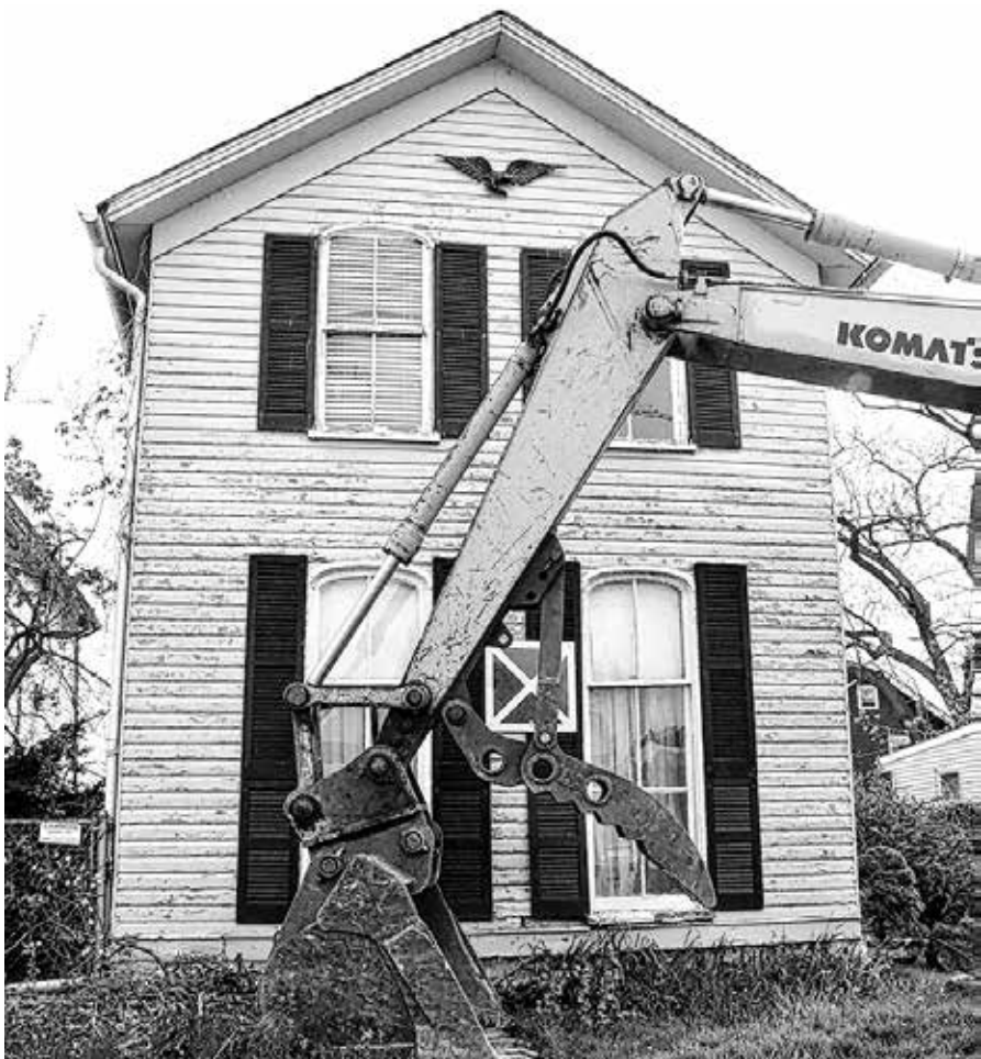
The house moments before the demolition started. The red box with a white X in it means the house is unsafe for humans. This is to warn people of rotted floors or unsafe wiring in case the police, firemen or someone else enters the property.
